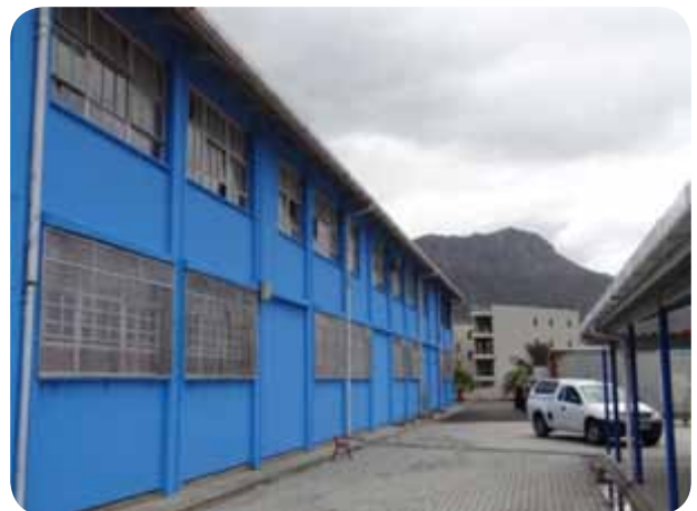
Refurbishment of Sentinel Primary School, Hout Bay
