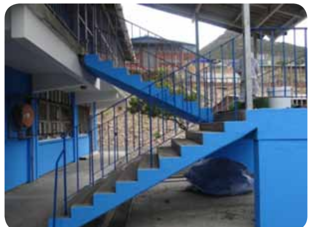
Refurbishment of Sentinel Primary School, Hout Bay
