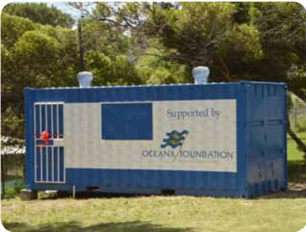
School feeding kitchen at Silikamva High School, Hout Bay
